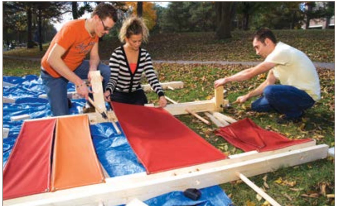
For a third-year project, BAS students designed and built outdoor dining pavilions, weaving food and architecture together. Students were encouraged to use found objects and recyclable materials.
